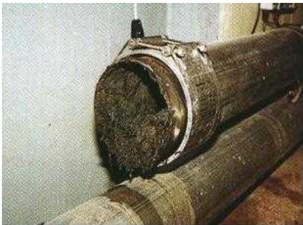
III.: Muddy water pipe without handling through the FLUID-LINER ®
